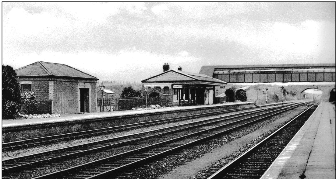
Figure 3: Photo of the former Ardley station and footbridge (former Bridge 42), taken from the western platform facing south towards the B430 overbridge (Bridge 41) 4
